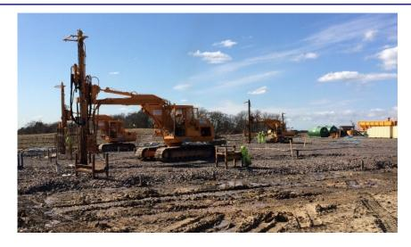
Contract to undertake shallow mine workings consolidation along the route of the M8 improvements being constructed by the Ferrovial Lagan JV in a DBFO contract for Transport Scotland.
